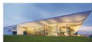
Lab - Italcementi Bergamo - General Contractor Impresa Pandini
